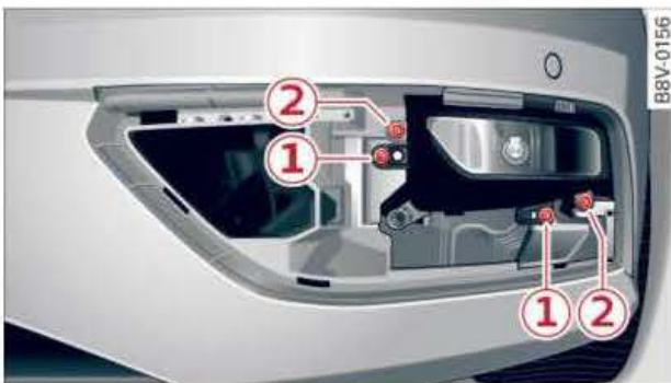
Fig. 288 Detail from front of vehicle, left side: Fog light
