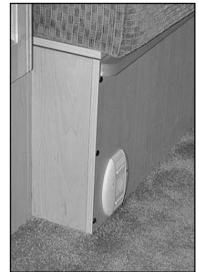
Picture F-P1A: L.P.G. leak detector, Versatile model.
