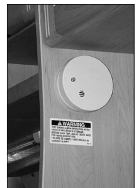
Picture F-P3A: Smoke detector, Versatile model.
