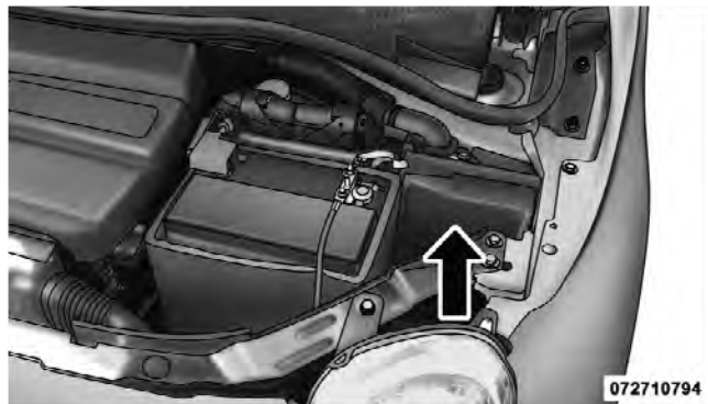
Front Distribution Unit
