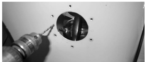
Figure 191: Carefully drill new holes
