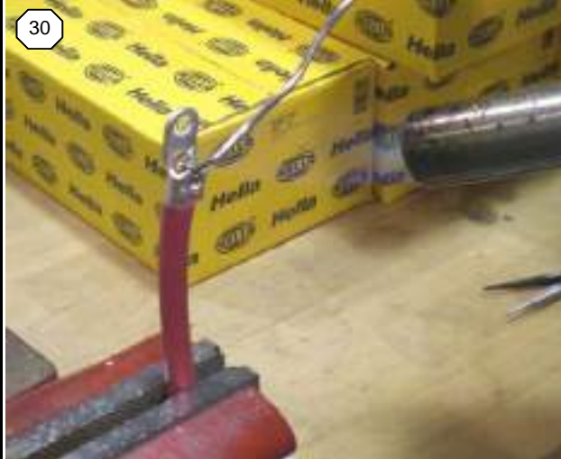
POSITION THE HEAT SHRINK AS SHOWN
