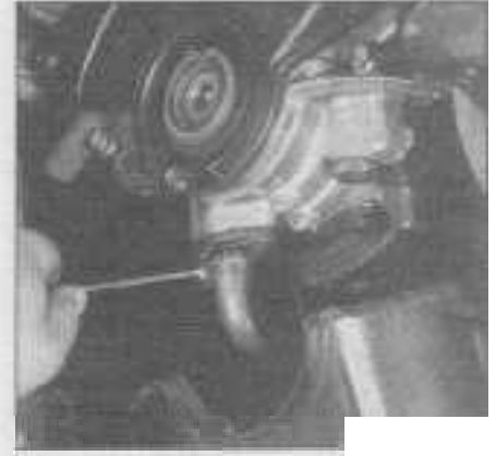
13.11a Lower the front of the oil pan to access the oil pump pick-up tube and remove the mounting bolts ...
