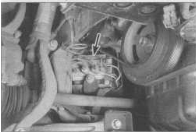
2.3 The Hydraulic Control Unit (arrow) is located below the power steering pump
