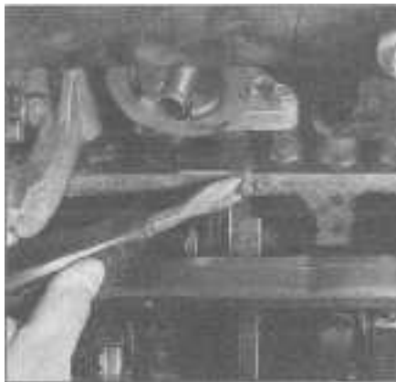
13.13a Thoroughly clean the oil pan and engine block gasket surfaces with a scraper to remove all traces of old gasket material
