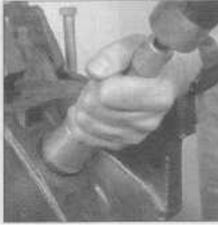
17.10 A large 1/2 drive socket on an extension can be used to drive the new core plugs into the block
