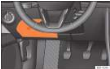
Fig. 104 On the dashboard on the driver side: lid of the fuse box.
